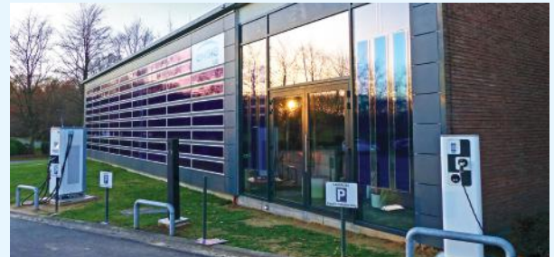
Building-integrated PV pilot project at ENGIE Laborelec in Belgium
