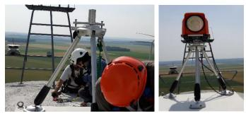
As well as installing the LIDAR equipment, Laborelec takes care of all the other aspects of the campaign, from the preparation of safety documentation to remote monitoring and data analysis.
