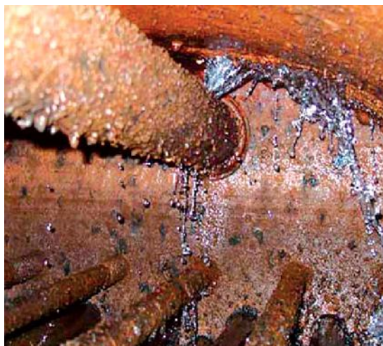
Corrosion of boiler pipes
