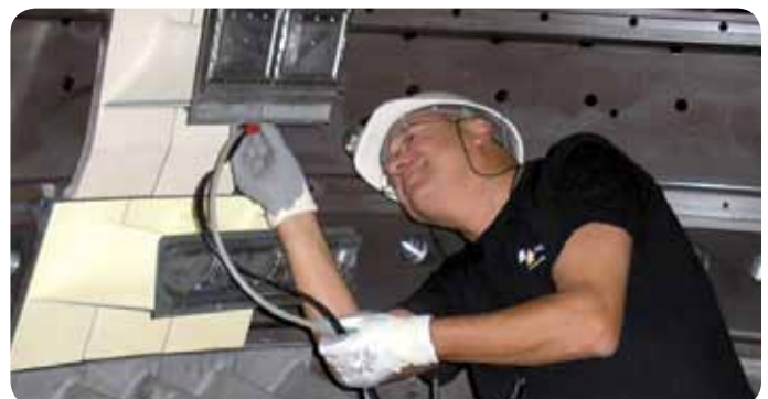
Using the F-SECT technology, Laborelec can assess the effect of burning syngas on a metallic coating underneath a ceramic layer.
