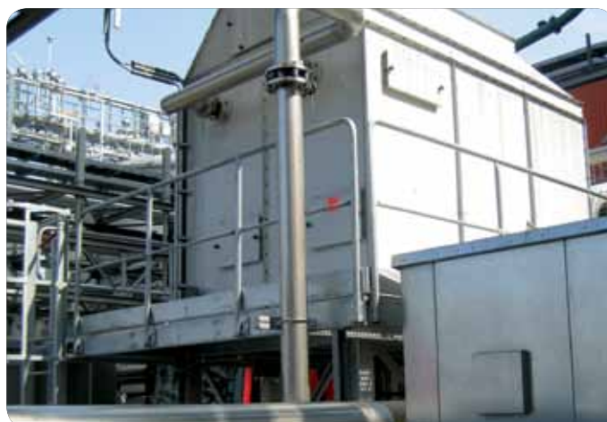
A chlorine dioxide dosing installation constantly feeds the circuit to disinfect the water and keep the Legionella growth under control.
