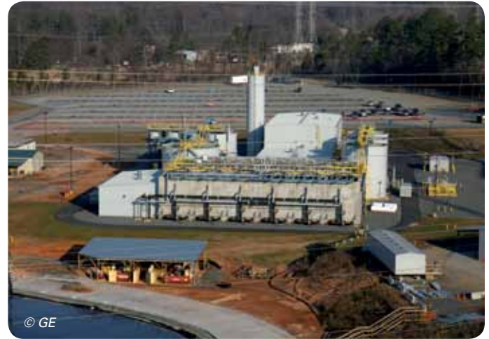
Tests with a pilot biological anaerobic FGD wastewater treatment system proved promising, although the engineering clearly needed optimization.
