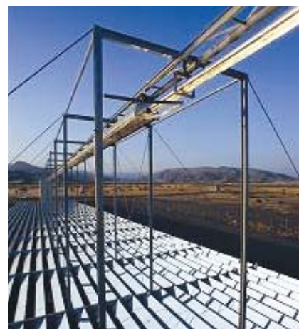
Laborelec will test the integration of thermal CSP technologies in a combined cycle gas turbine.
