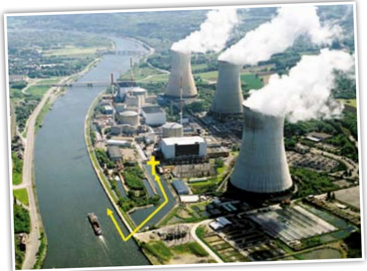
Thanks to the infrasonic fence, 80% of the fish population safely pass the water intakes at the Tihange Nuclear Power Plant.
