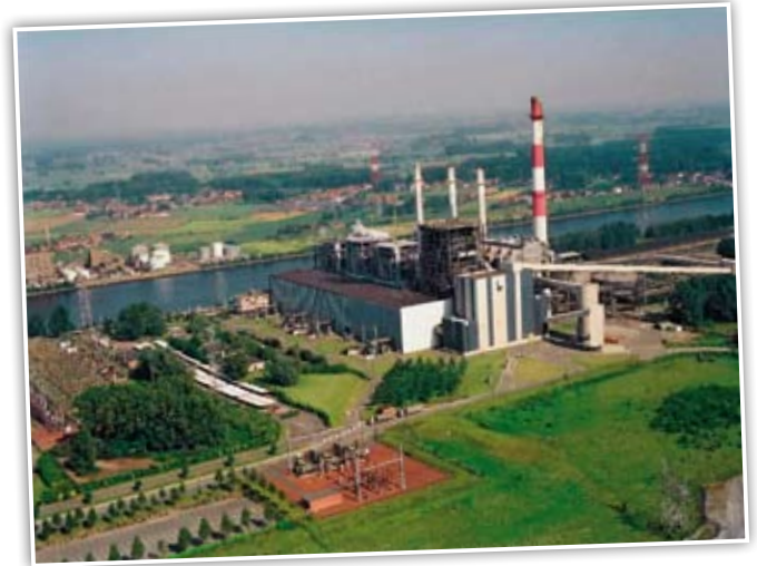
By 2011, Rodenhuize 4 will be fired entirely with biomass.
