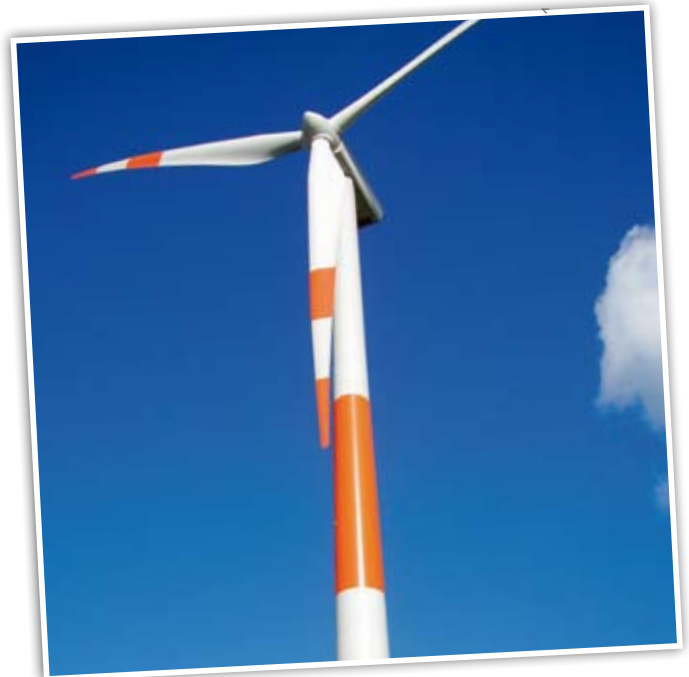
Vibration monitoring is essential for efficient maintenance planning of wind turbines.
