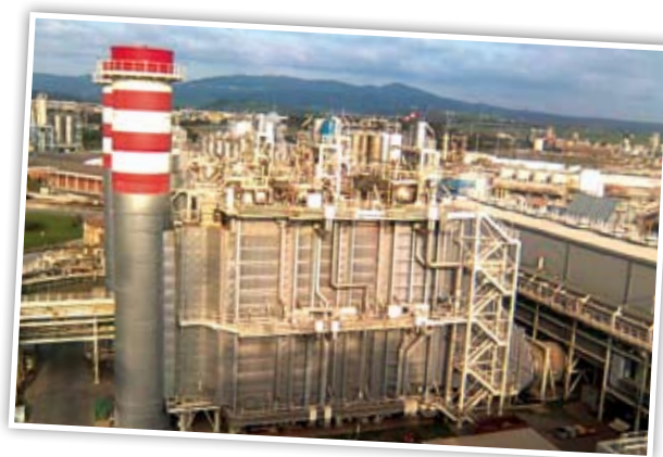
The service agreement also covers interventions during or after an unexpected issue, such as a broken turbine blade.
